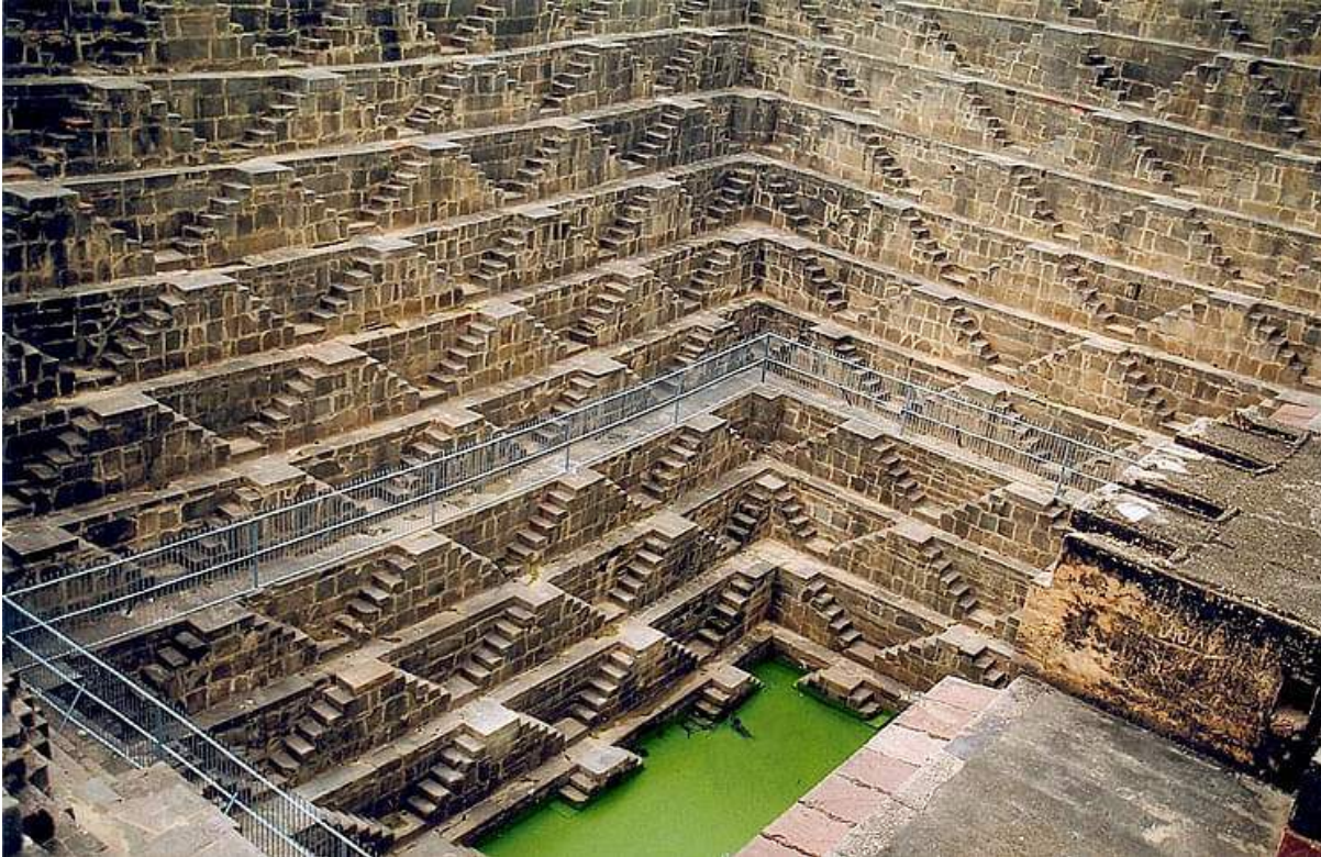
Figure 1: A jhalara showing clear steps to reach water at different levels.
