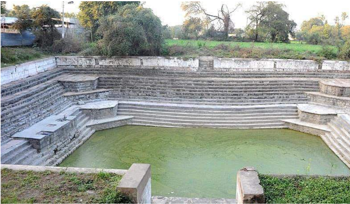
Figure 5: A kund: traditionally made from lime and ash in some sandy regions of India.
