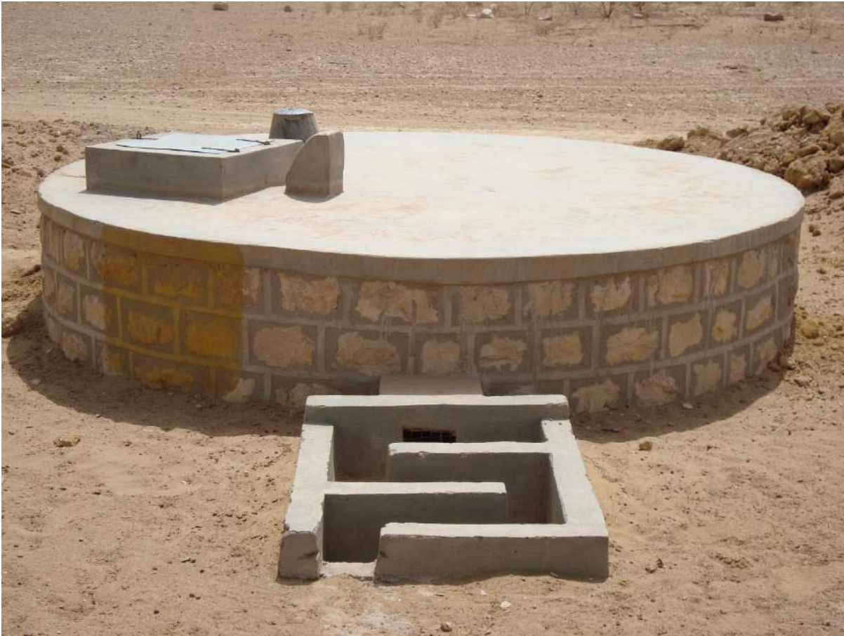
Figure 3: The cover of a cylindrical taanka water capture and storage system.
